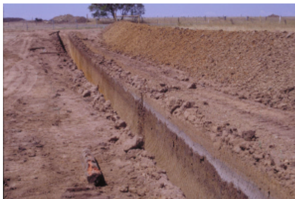
Trenched section at SW99 showing disappearance of A2 away from drainage line
